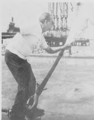
Above and beside: Fred Linde and John Sine of National Foam are checking the pump capacity of a fire truck.
